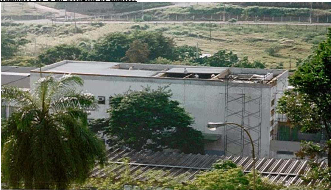
Figure 7. The New Roof of the Reactor Building
