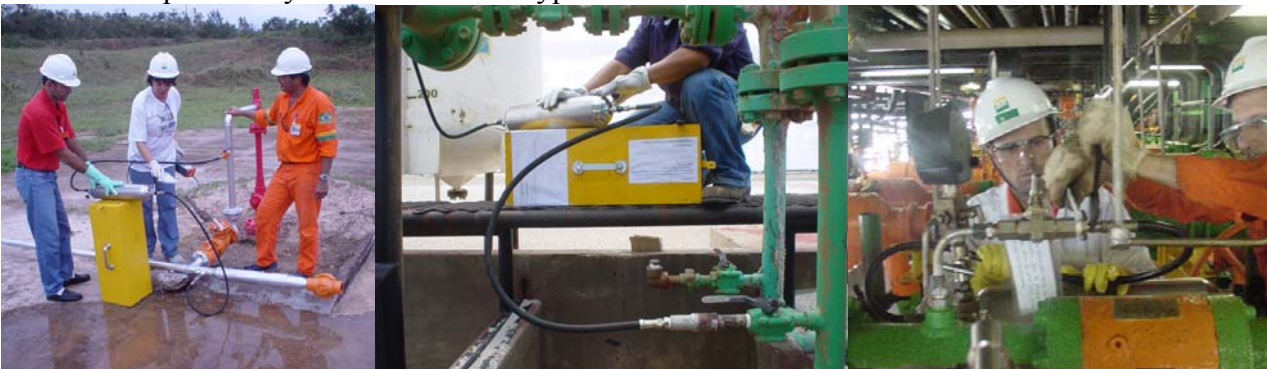
Figure 08 – scheme of the bypass in the field.
