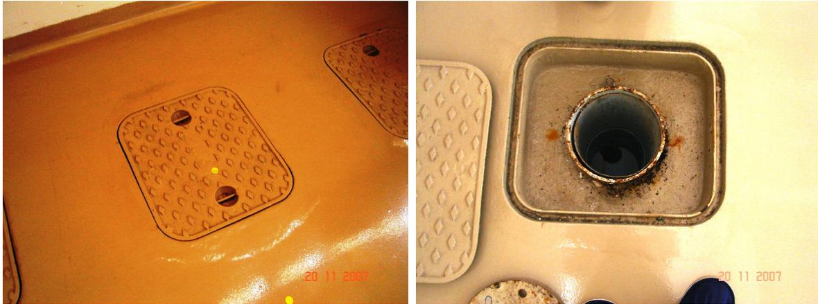
Figure 5. Well for storage of irradiated fuel elements
