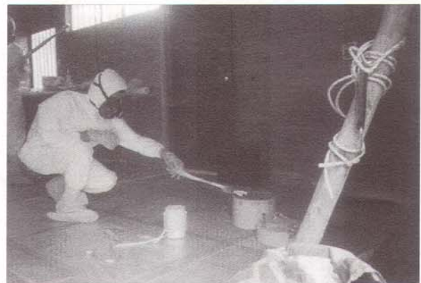
Fig. 6. Transferring a capsule to the final lead shield.
